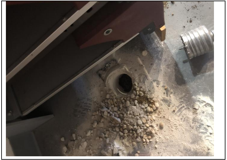
2. View of WHS630-1 sample area.
