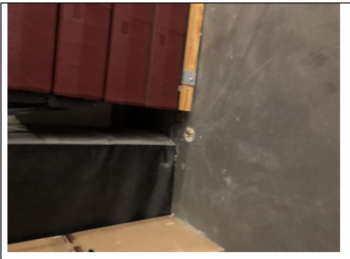
5. View of WHS630-7 sample area
